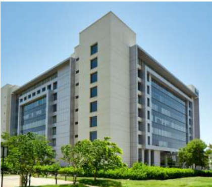
Embassy TechZone Pune (5.5 msf)
