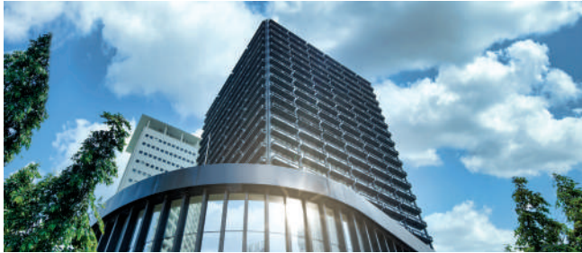
Express Towers Mumbai (0.5 msf)
