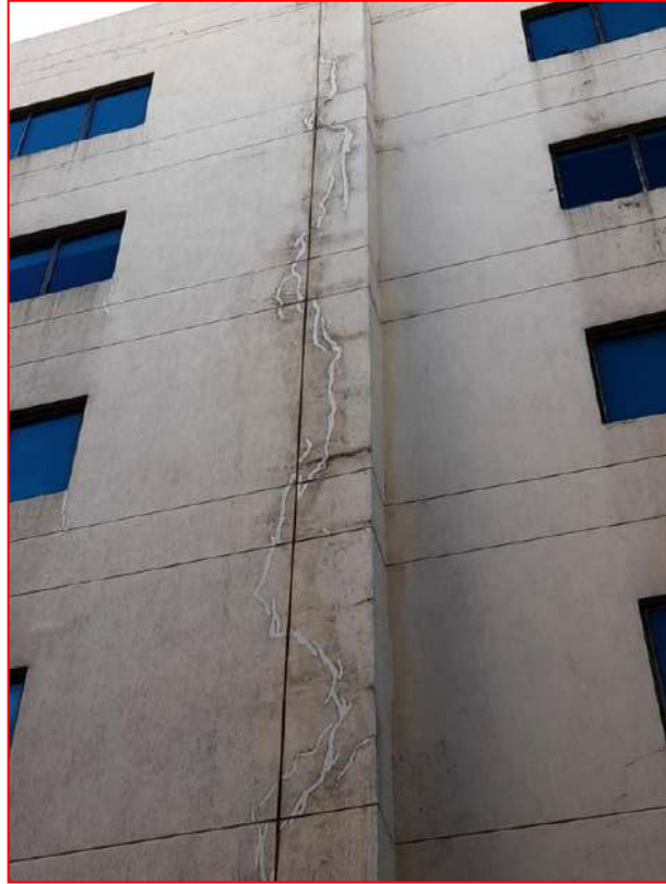
Cracks in plaster and filled sealant.
