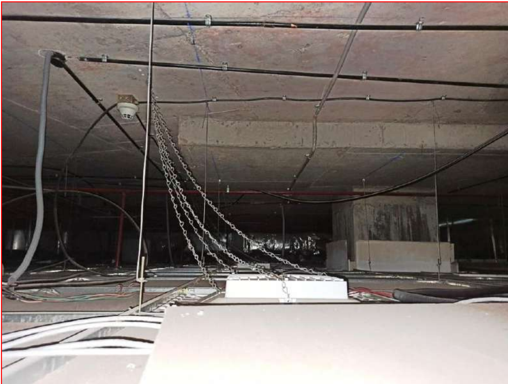
View of ceiling Slab, Column & Column cap which is in satisfactory condition.
