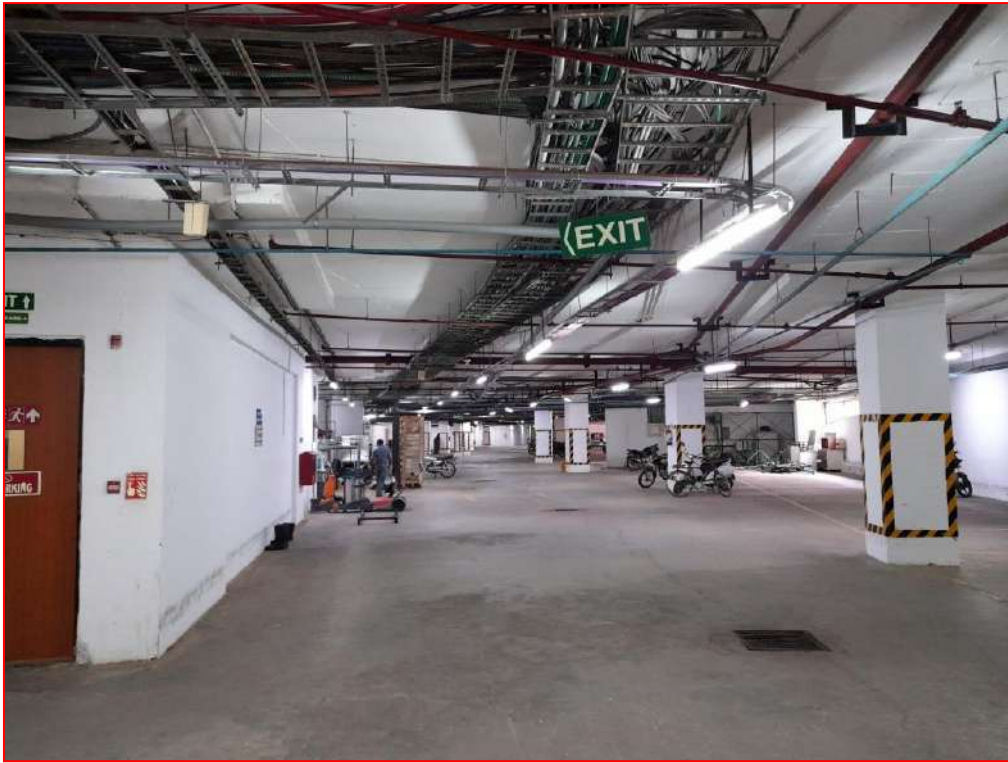
View of basement
