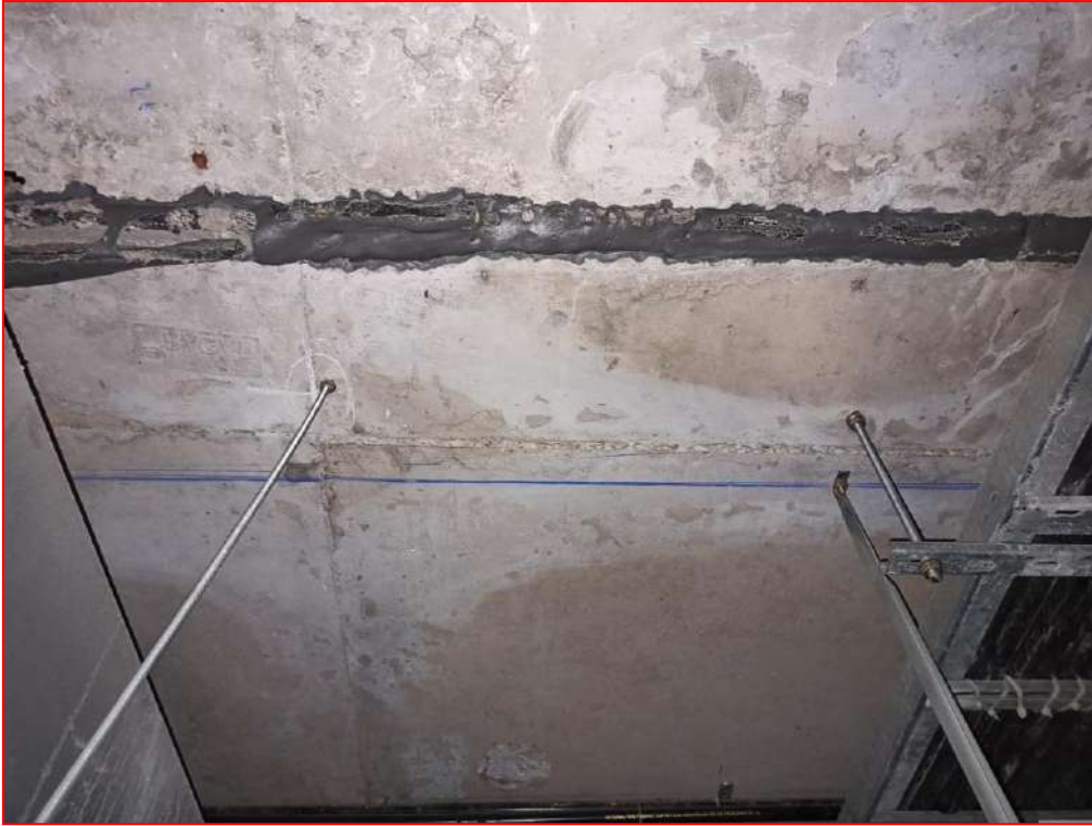
View of Expansion joint was repair with Chemicals & filler materials.
