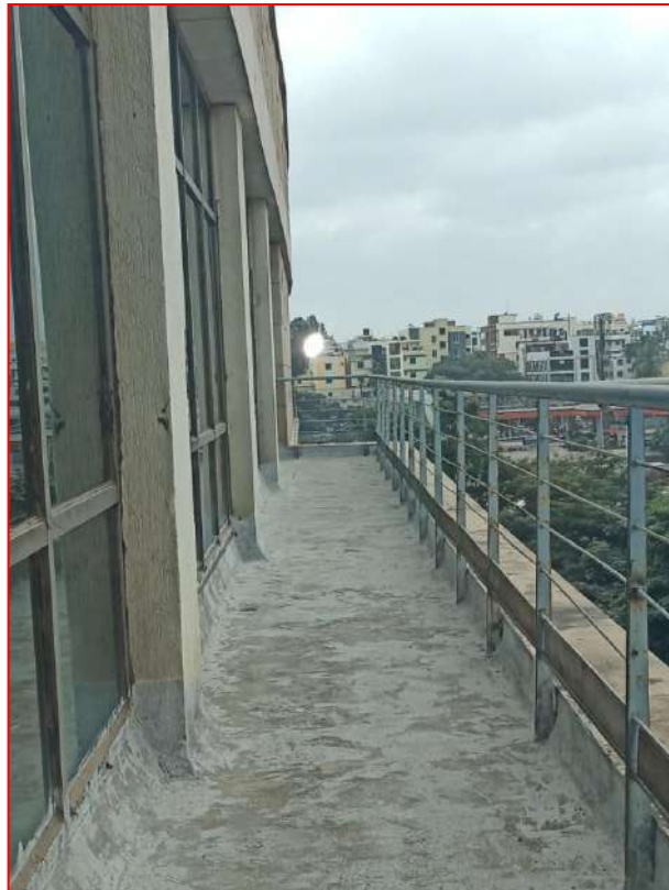
Chemical water proof coating was done on open balcony floor surface.
