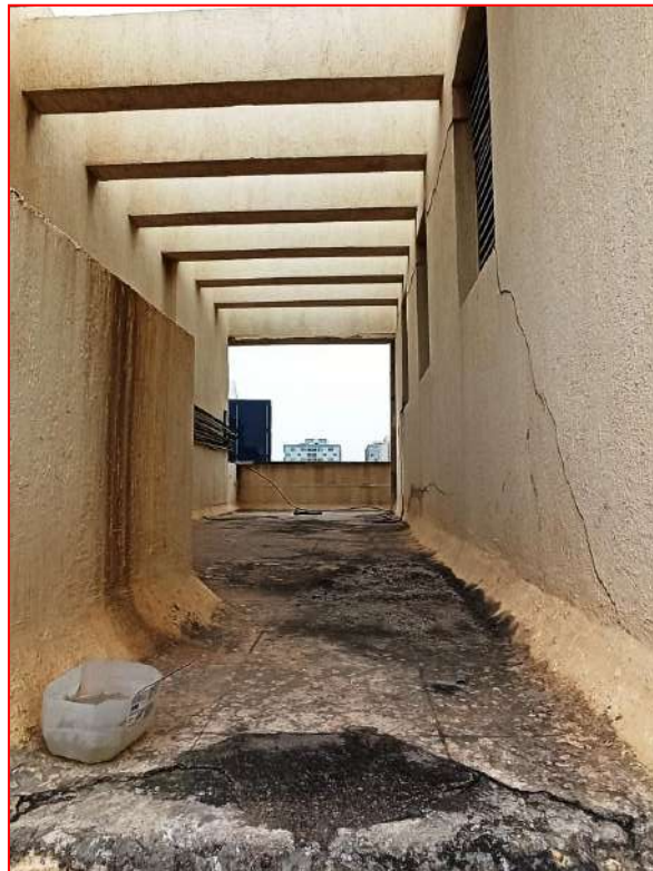
Open terrace at 4 th floor: View of discolored and damaged IPS with masonry cracks on wall.
