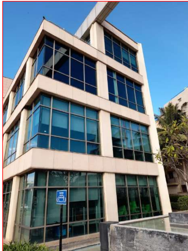
Side view of Building consist Glass cladding & stone cladding.
