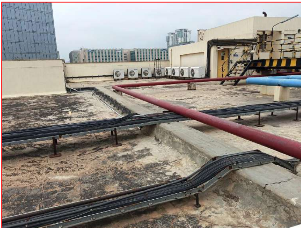
View of various service pipe lines and electrical cables run on terrace surface with the support of concrete pedestal and GI cable tray. Bund wall observed with cracks.
