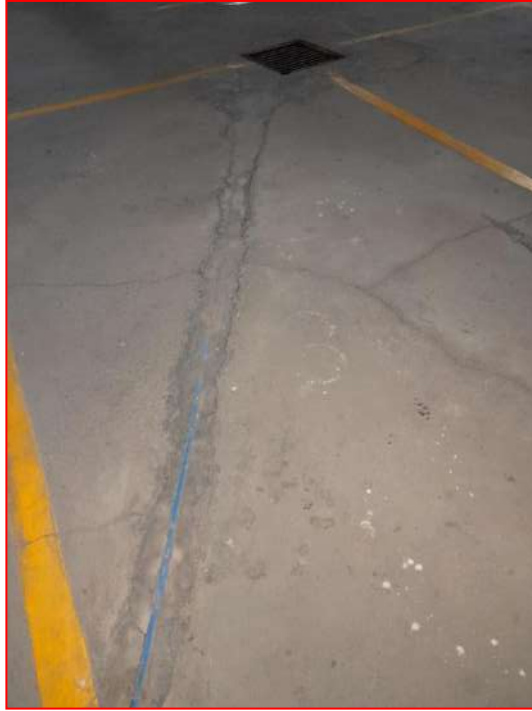
PVC drains pipes fixed inside flooring.
