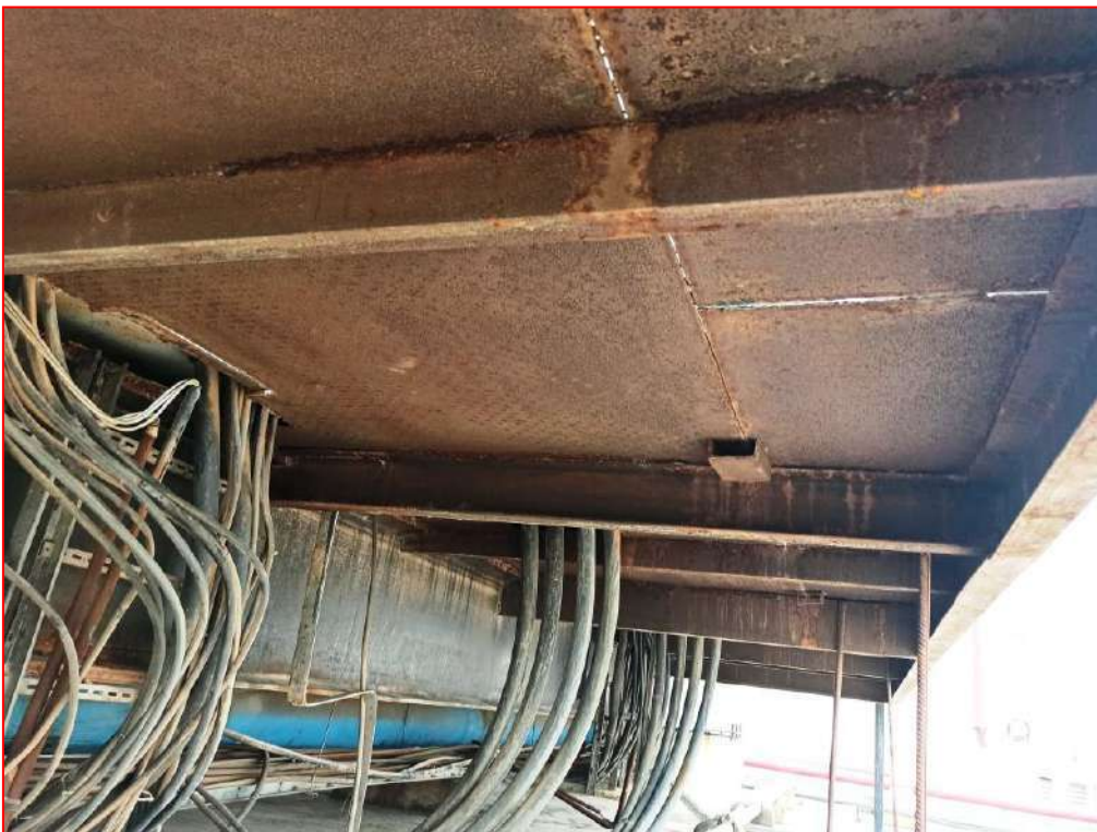
Close view reveals Structural steel members and MS chequered plate were found corroded of chiller platform.
