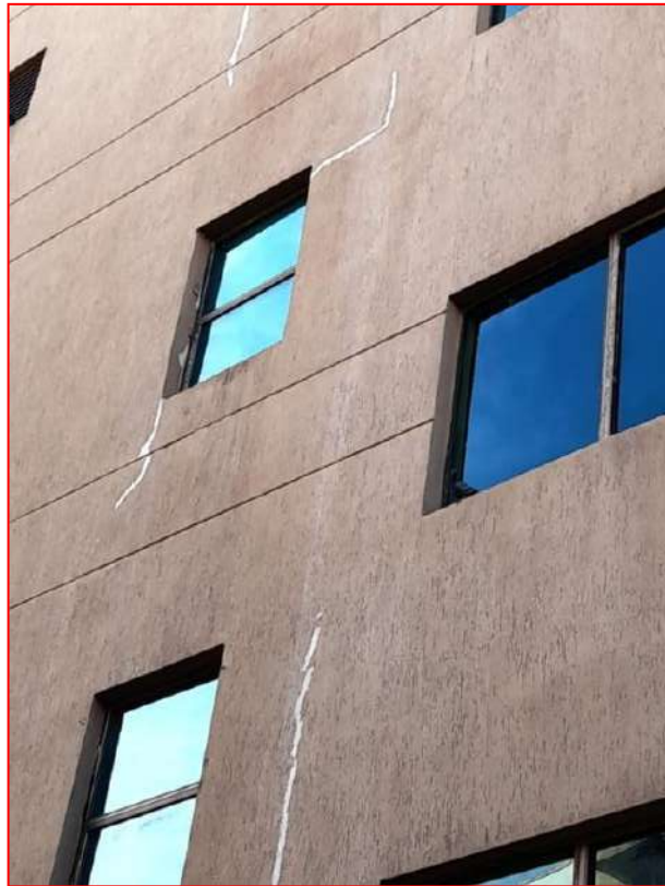
Cracks in plaster and filled sealant.
