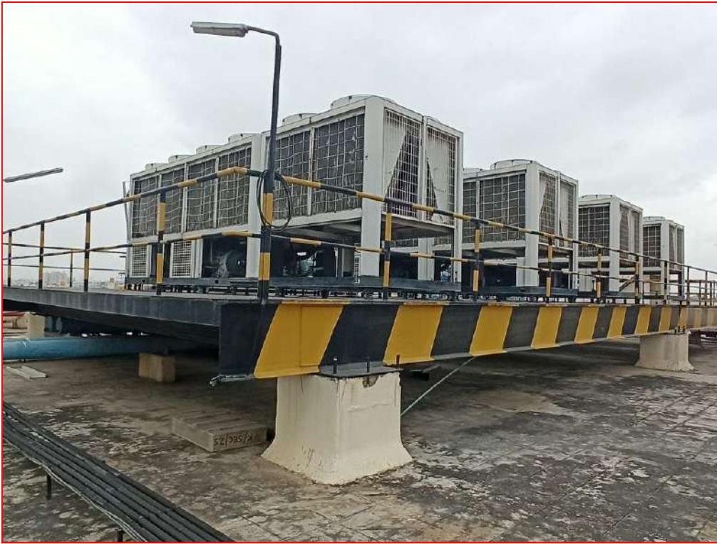
View of structural steel chiller platform.
