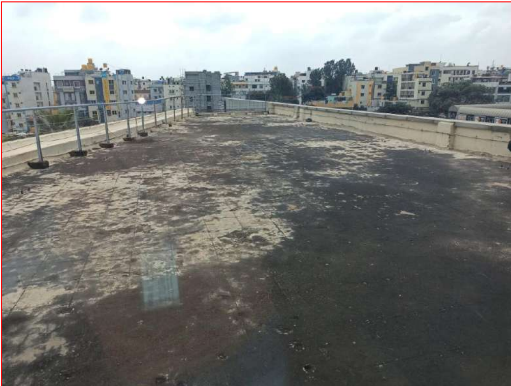
4 th floor level open terrace observed with major discoloration due to ingress of rain water.
