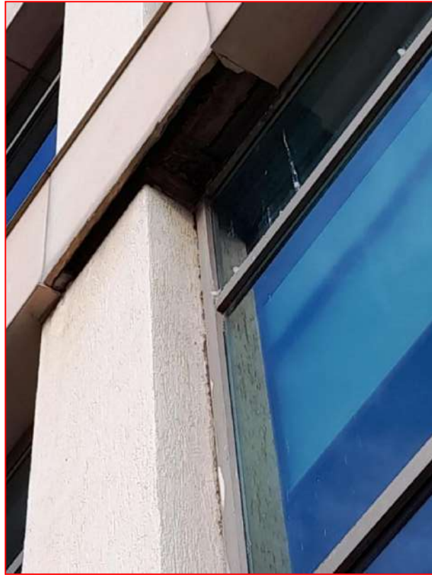
Stone cladding along the external walls are debonded and cracked.
