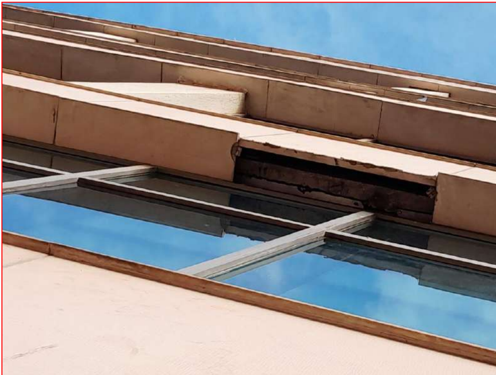
Stone cladding along the external walls are debonded and cracked.
