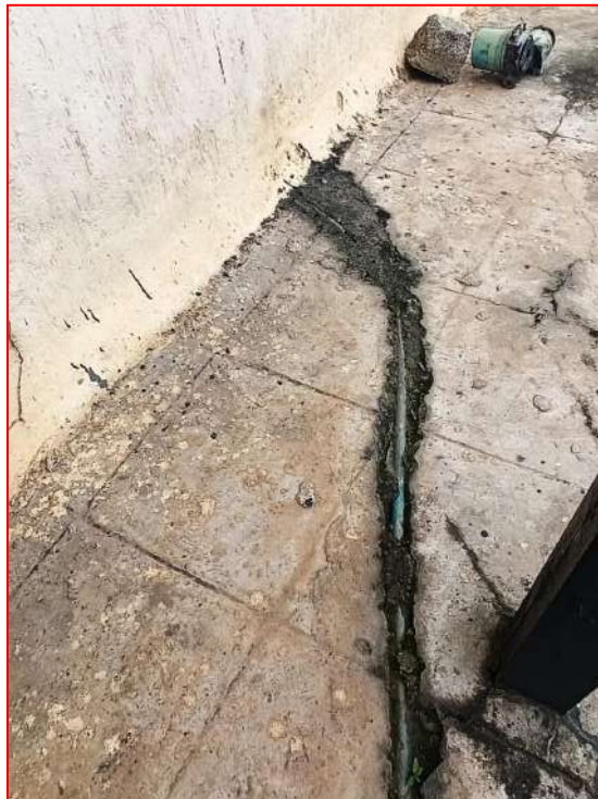
Pipe is embedded in the IPS but without proper cover over it. Thus exposing the waterproofing.
