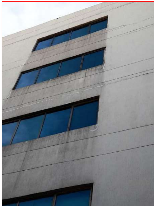
Discoloration marks were observed over the external wall below windows.
