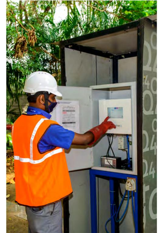
▶ COD/BOD sensor installed at the STP in Quadron, Pune. This provides water parameters online and helps avoid fines for exceeding permissible limits for discharge. The data generated also sheds light on opportunities to improve our use of STP water, thus enhancing water efficiency.
